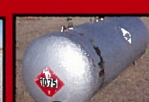
500 GAL PROPANE TANK
